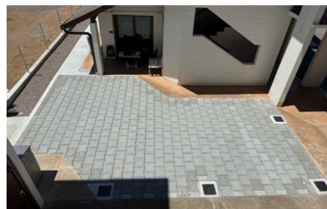
View from above of the newly completed courtyard. An observation that has been made is that this improvement may have abated the flies presence in the area and social halls.
