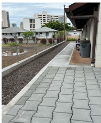
Long view of the sidewalk extension pavers, provide ample space for rolling walkers, wheelchairs and strollers
